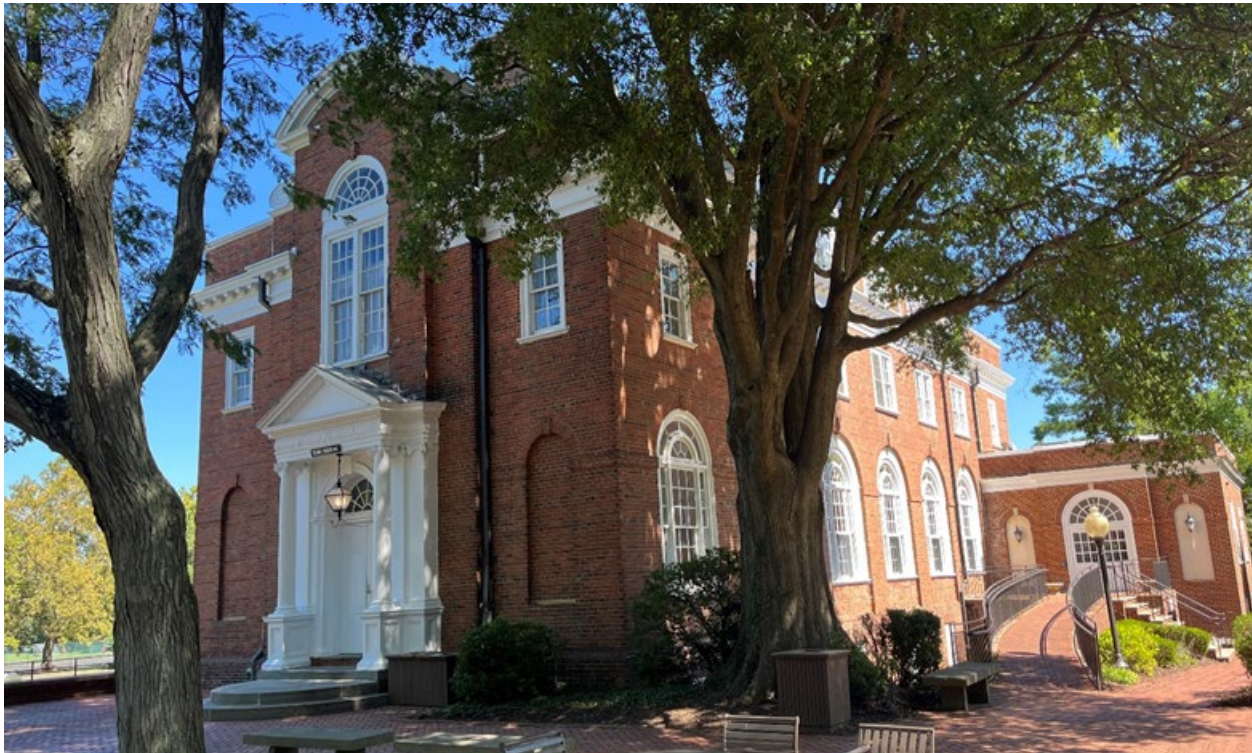
Figure 51: Southwest elevation of Randall Hall, looking north. EHT Traceries, August 2023.
