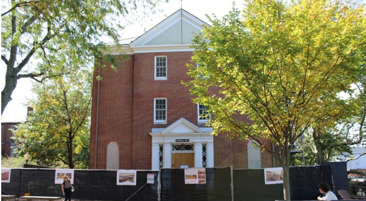
Figure 55: Northeast elevation of Campbell Hall, looking southwest. EHT Tracerics, October 2023.
