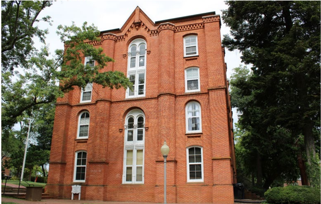
Figure 43: Southeast elevation of Pinkney Hall, looking northwest. EHT Traceries , August 2023.
