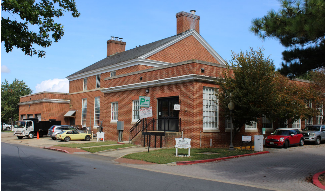
Figure 54: Southwest and partial southeast elevations of the Heating Plant and Printing Shop, looking north. EHT Traceries, October 2023.
