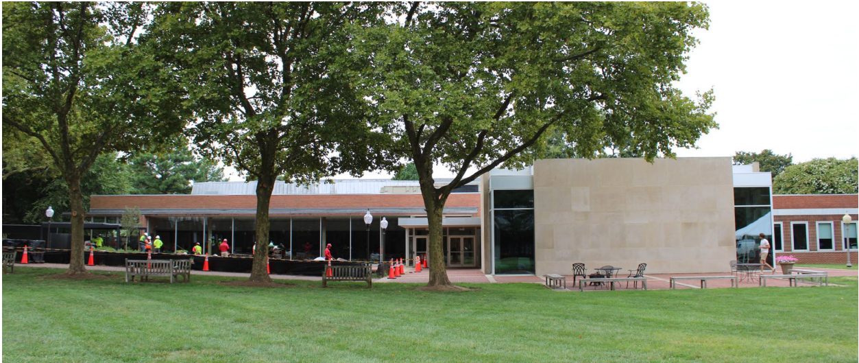
Figure 48: East corner of Key Memorial Hall, looking southwest. EHT Tracerics, August 2023.
